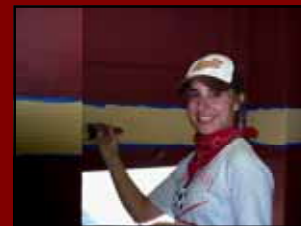
Several summer mission teams helped with renovations and community improvement projects.
